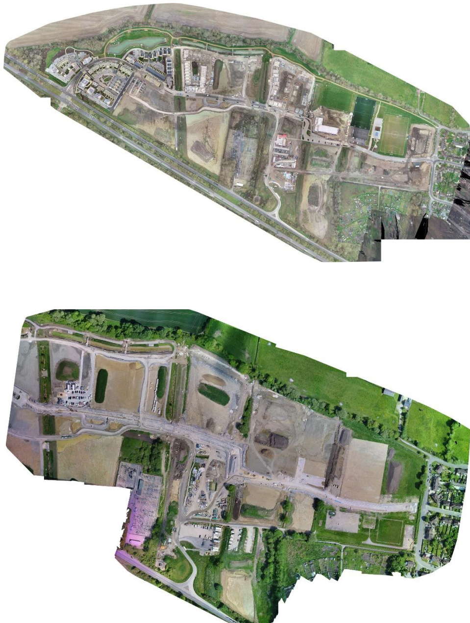
Figure 4. Construction Phase Aerials, 2017 (top) and 2020 (bottom), Barton Park, Development, Oxford, Tree Frontiers
