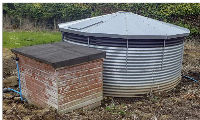
Covered borehole water storage tank.
