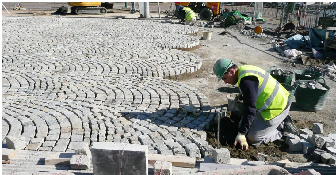
Fan tail pattern being laid using a rigid system at Castle Square in Caernarfon, a rare use of Welsh Granite.
