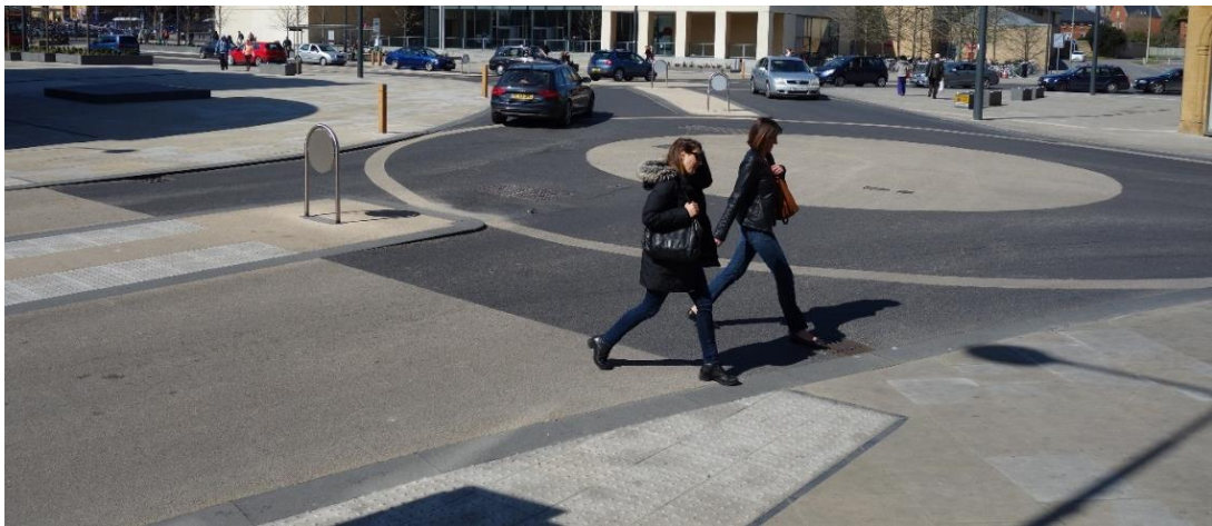
Frideswide Square, Oxford showing a roundel, courtesy crossing and central median with minimal formal highway infrastructure. The scheme includes three roundels which replaced a very busy and intrusive series of traffic lights.
